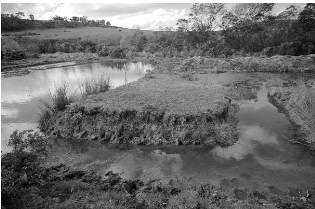
Plate 4. An example of a settling pond with baffles
