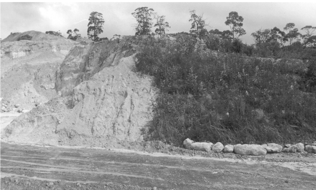
Plate 8. Example of the stabilisation of erosion by vegetation
