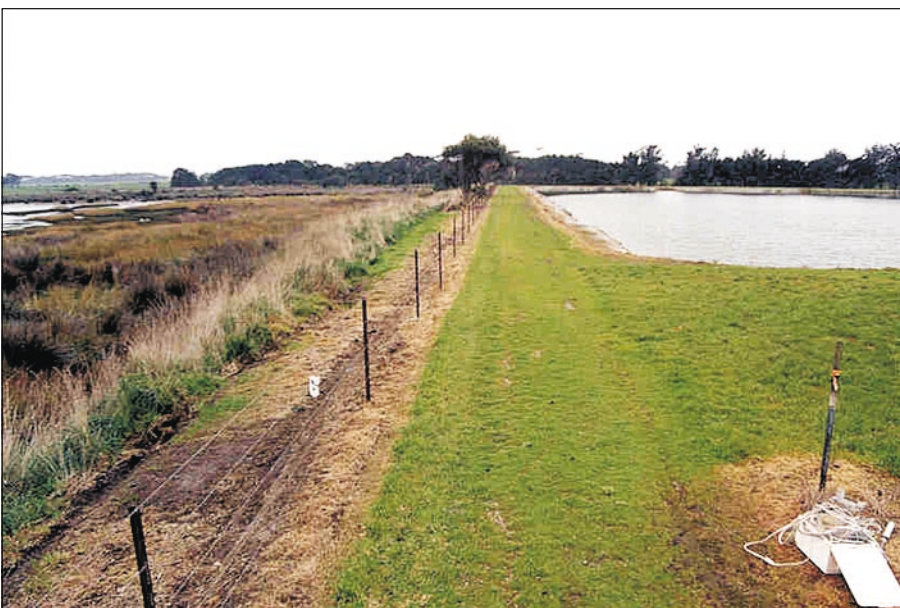
Plate 1. Lagoons constructed on tidal marsh deposits in the northwest corner of the site.
