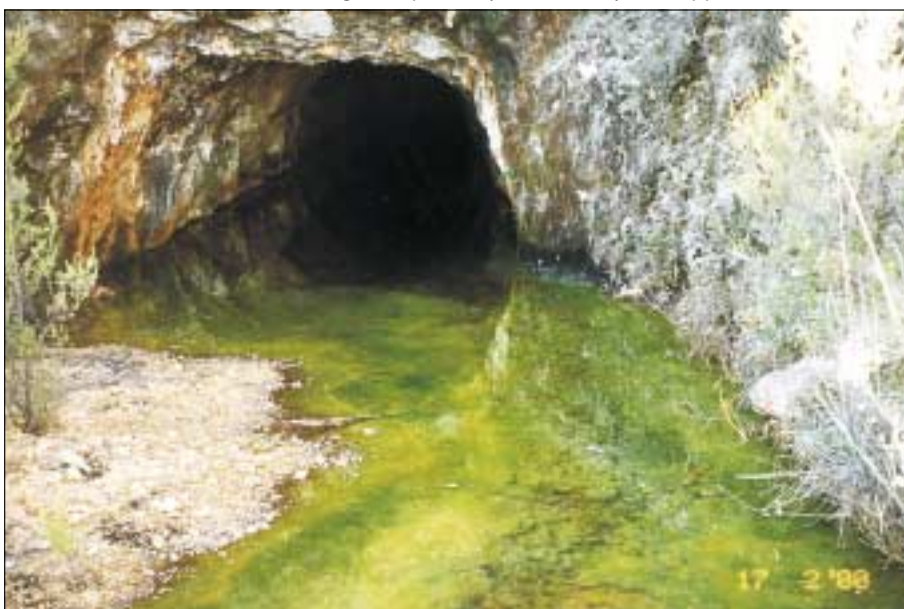
Plate 3. Acid drainage discharge from Mt Bischoff tin mine adit
