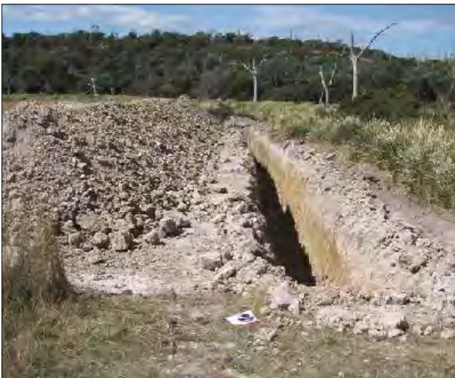
Costean at Rushy Lagoon showing topsoil and gravel stockpiles.
