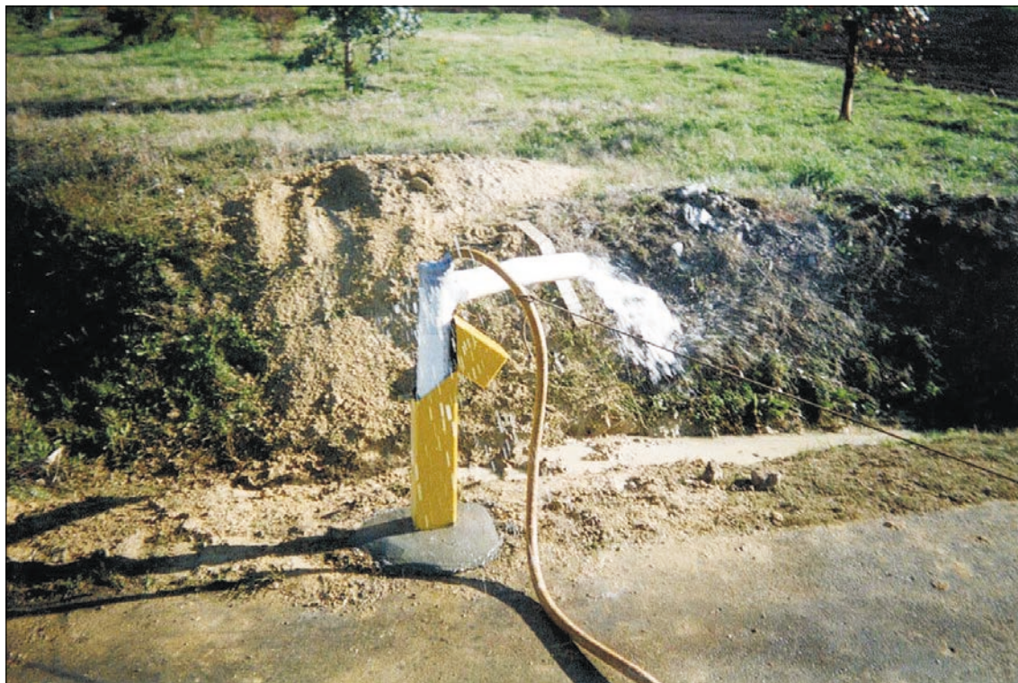
Plate 5 Developing bore hole JS2001/2.
