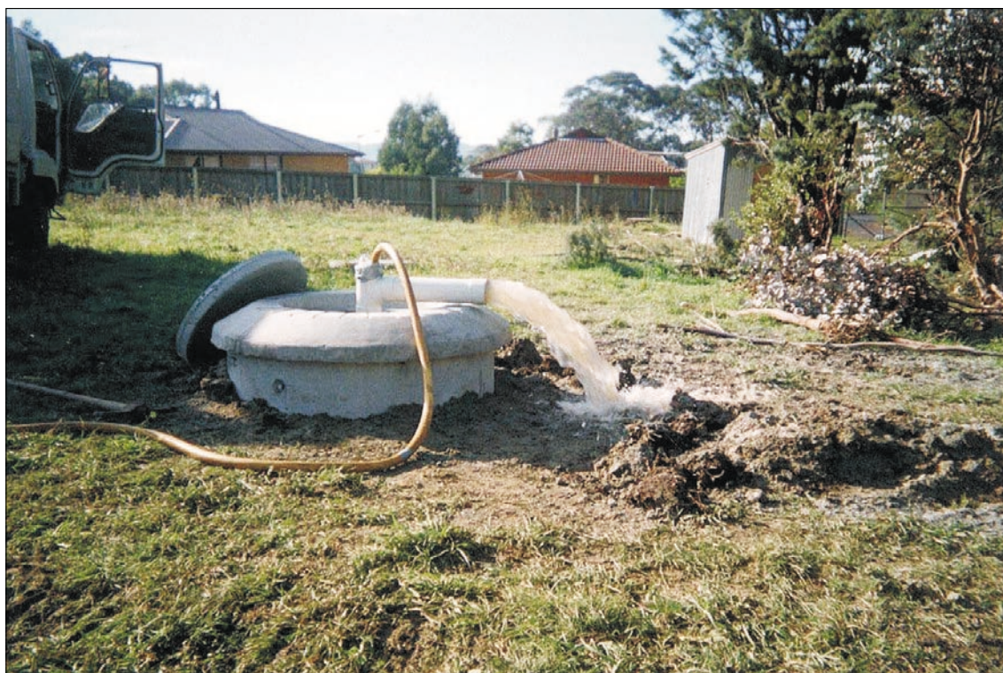
Plate 6 Developing bore hole CS2001/1. Note discolouration of water compared to Plates 4 and 5.
