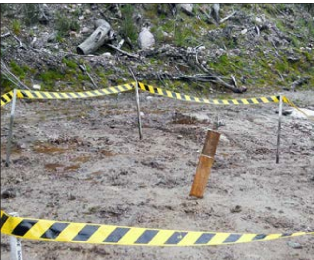
Three attempts to seal hole with eventual success at great cost. Note no solid secure collar.
