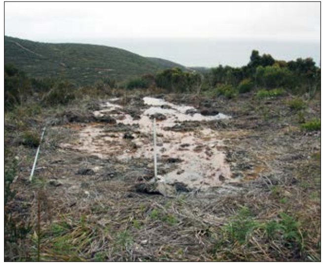
Attempts to seal hole failed because of poor collar.
