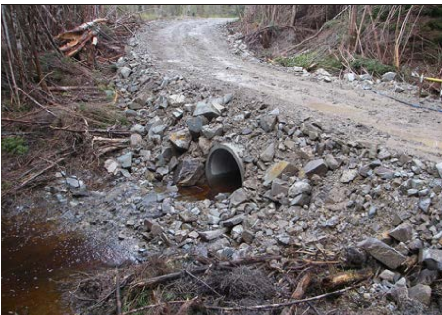
Well constructed concrete pipe culvert.
