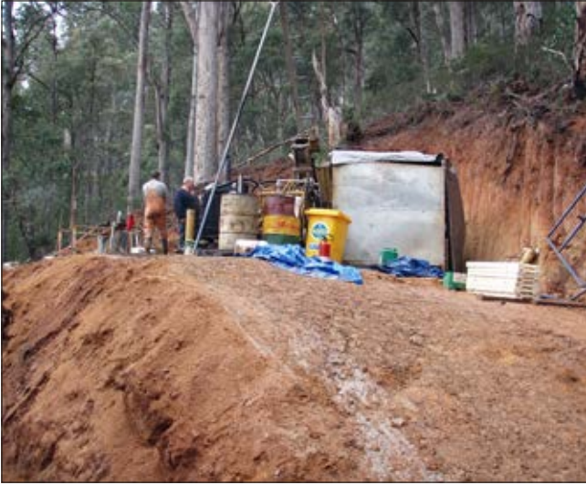
Drill site rehabilitation at Lorinna — July 2007
