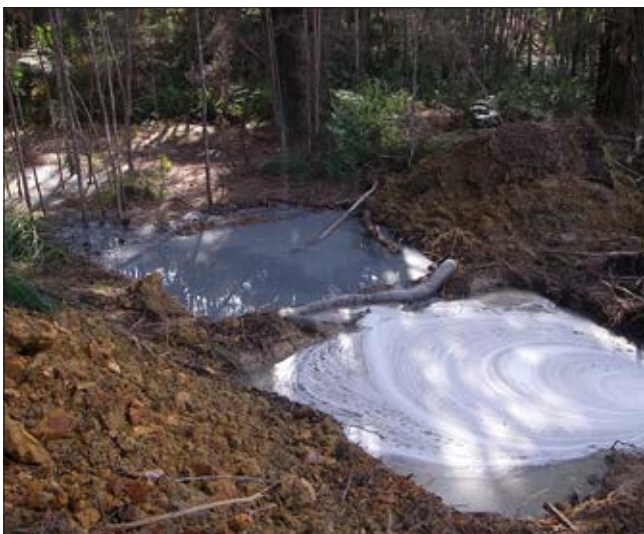
Dual excavated sump (above) and triple excavated sump (right).
