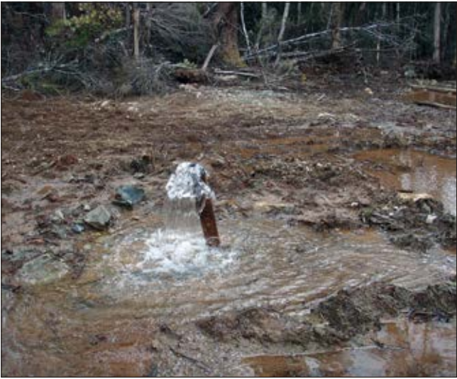
Drill hole making water.
