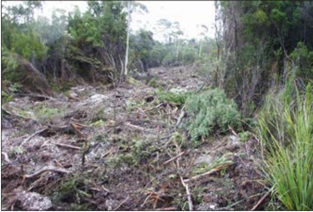
Track rehabilitation using stored topsoil and vegetation — July 2001.
