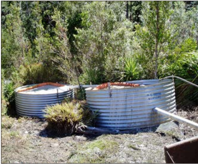
Excellent example of remote area above ground sumps — note oil absorbent mat and sausage.
