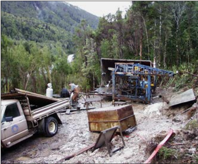
Drill site rehabilitation adjacent to Jukes Road — July 2001
