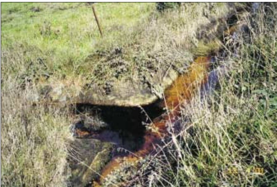
Plate 2. Acid drainage discharge from disturbance of acid sulphate soil at Mella, northwest Tasmania
