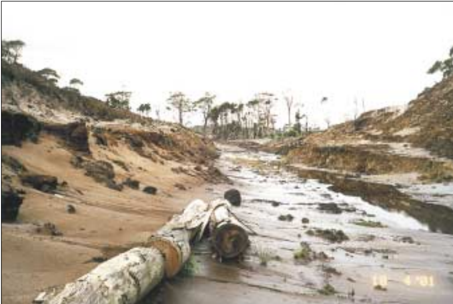
Plate 5. Potential acid sulphate soil disturbance from a channel excavation, northwest Tasmania
