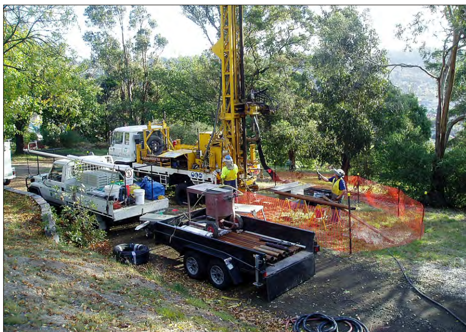
Plate 5 Drilling set up at drill hole LV_IBH1_2005, April 2005.
