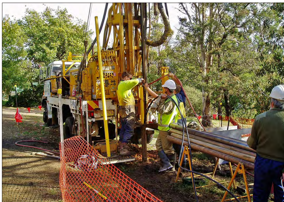
Plate 6 Inclinometer being installed in drill hole LV_IBH1_2005, April 2005.
